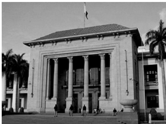
Building of Provincial Assembly of the Punjab, Lahore
